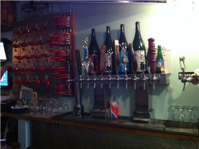
22 Tap "Flux Capacitor" allows each beer to be served at correct pressure and with one of 5 gas mixes as appropriate.
